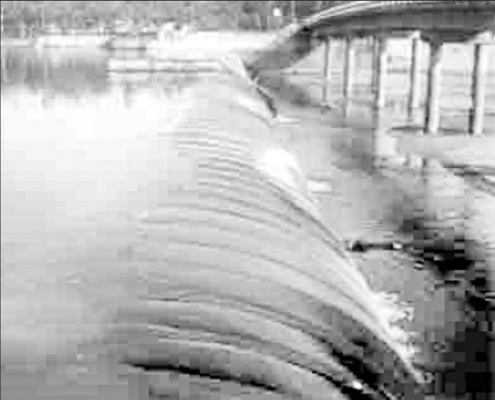
Water flowing over the rubber dam at Jamirakanda (left) being taken to IRRI-Boro lands through a canal.
