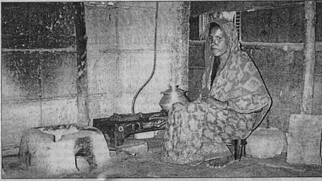
A housewife of Dainna village in Tangail Sadar upazila cooking food by bio-gas produced in her plant. Local people installed bio-gas plants on personal initiative and changed their lives rapidly.
