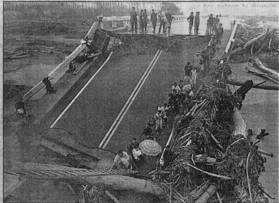
Residents from Banugaw village climb down using a rope to cross a fallen concrete bridge in the eastern Philippine town of General Nakar yesterday. The bridge was knocked down by the floating logs brought down by the floods panned by a storm that hit the eastern part of the Philippines. The death toll from the storm has risen above 150 as the towns of General Nakar, Infanta and Real are isolated by the toppling of their bridges.
