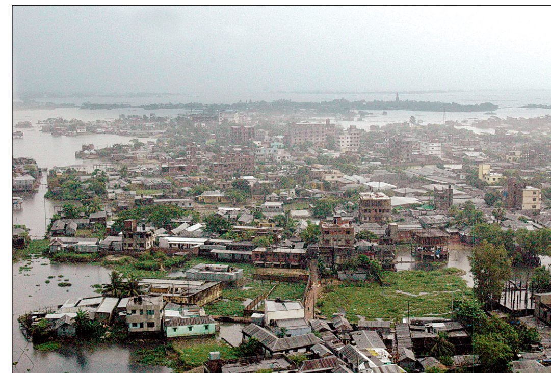
A bird's eye view of the eastern part of Dhaka where the Eastern Bypass will be built.
