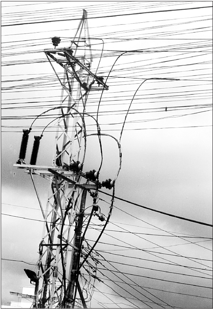
A power distribution post in Old Dhaka with illegal power lines drawn in every direction cause great loss to PDB and Desa.
