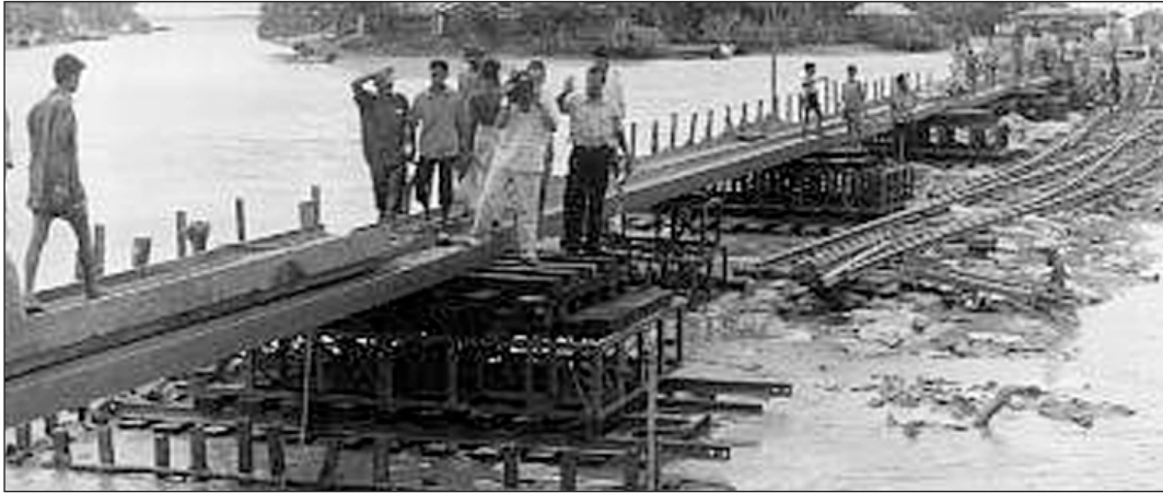
A temporary bridge is being erected at the breached portion of the Trimohoni-Balashi rail track. The photo was taken on Friday.
