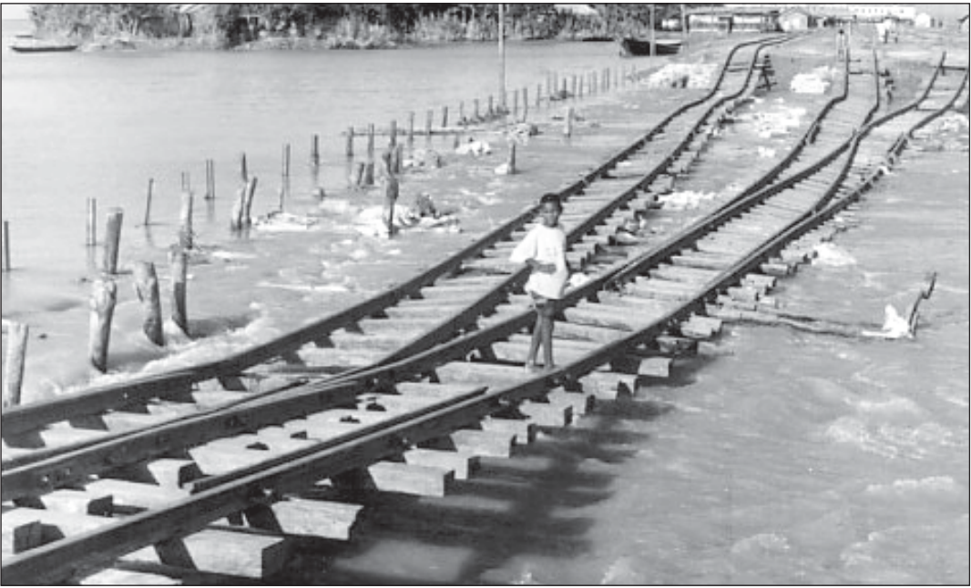
Over 1000 feet rail tracks between Trimohoni and Teestamukh Ghat in Gaibandha are virtually hanging as the soil underneath has been washed away by flood.
