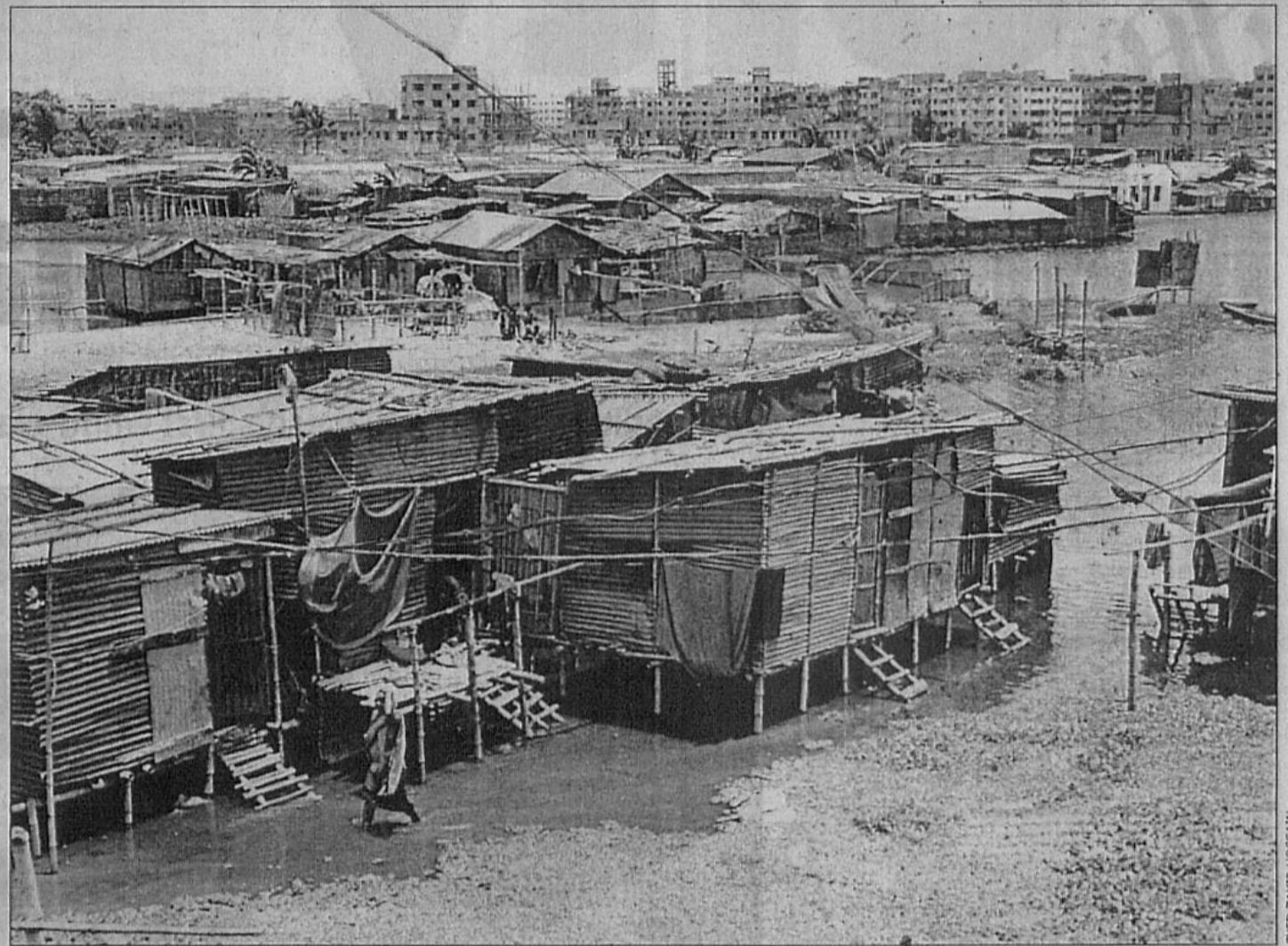
Waterlogged Rayer Bazar in the DND dam area.
