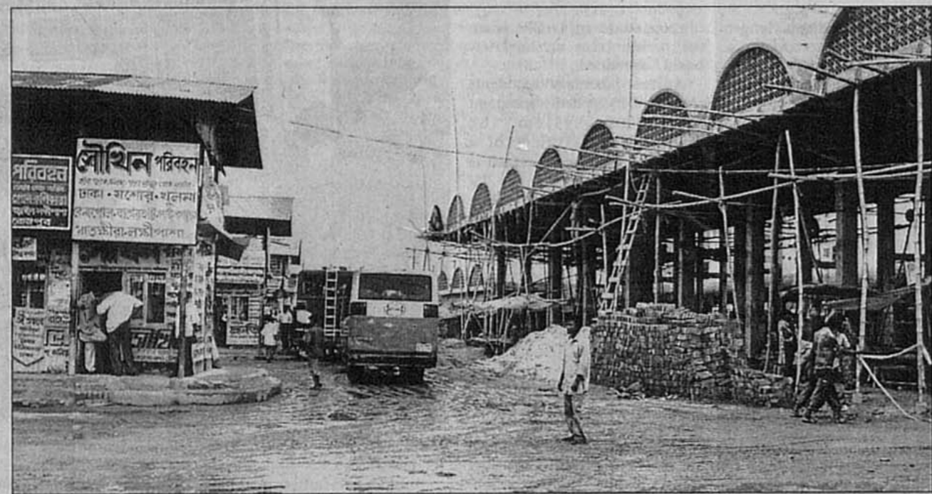
Development work in progress at Gabtoli terminal.
