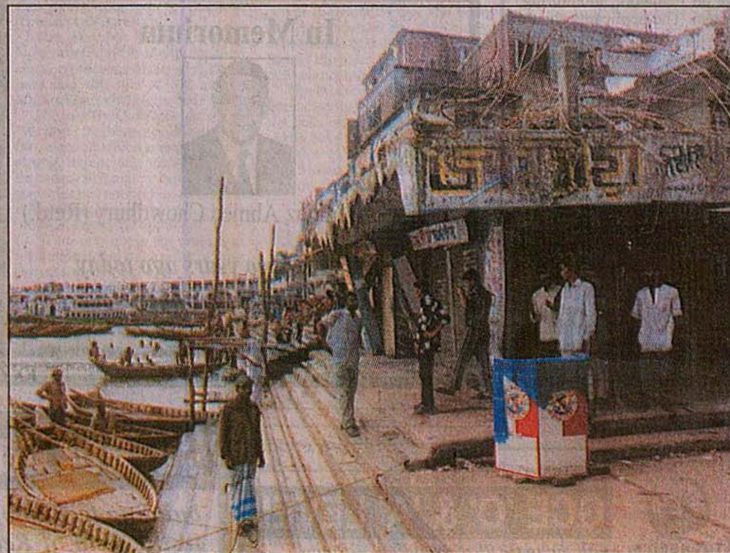
A recent drive against encroachers on Buriganga left this Zila Parishad Market built by government funds untouched although other illegal structures beside it were knocked down.
