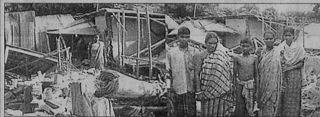
Families of Chinta Moni Bala and Parimal in front of their demolished houses, snapped on Saturday
