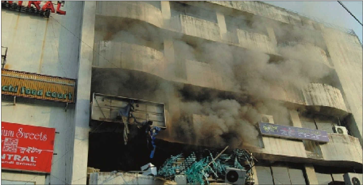
Smoke billows from a dental surgery in Dhanmondi as an explosion shattered its windowpanes and injured five people, setting the second floor of the building on fire yesterday.
