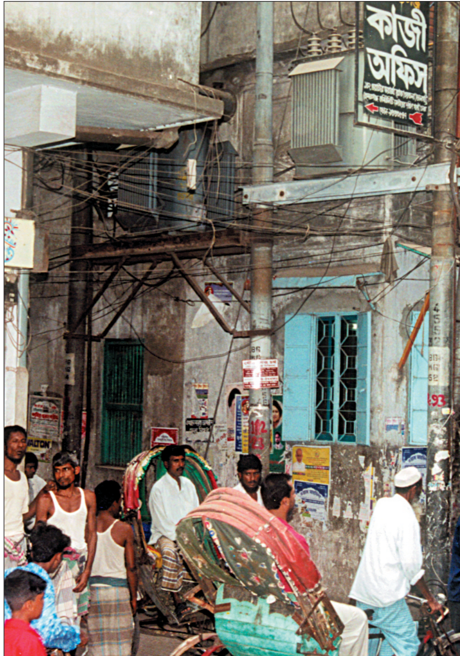
Three transformers dangerously close to buildings at Topkhana (left top), Lalbagh (bottom) and Rahamatganj (right).
