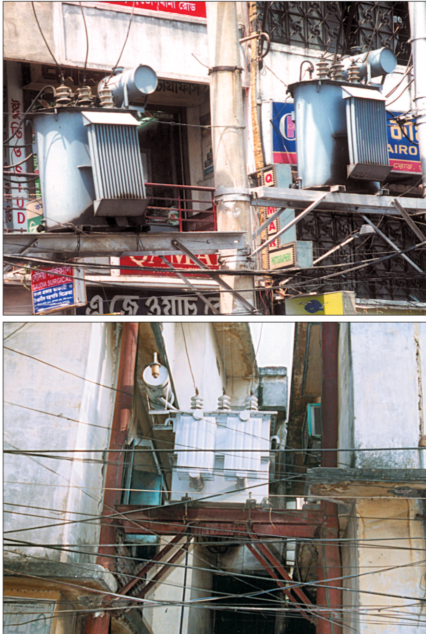
Three transformers dangerously close to buildings at Topkhana (left top), Lalbagh (bottom) and Rahamatganj (right).
