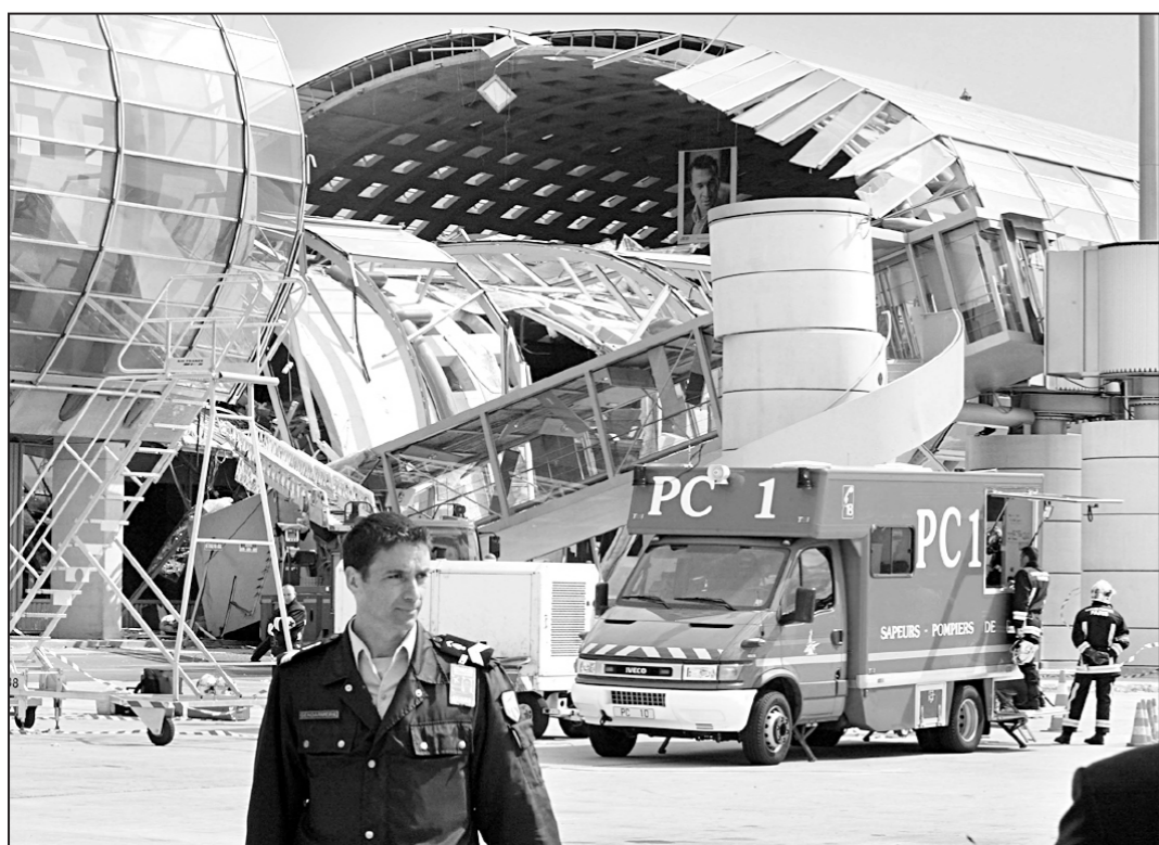
Emergency services work by the collapsed footway of the new terminal 2E at Roissy airport, outside Paris yesterday. Six people, including three police officers, were killed and at least three others were injured when heavy slabs of concrete from a roof crashed onto a boarding footway which in turn collapsed onto airport service vehicles parked below at Charles de Gaulle airport in France.
