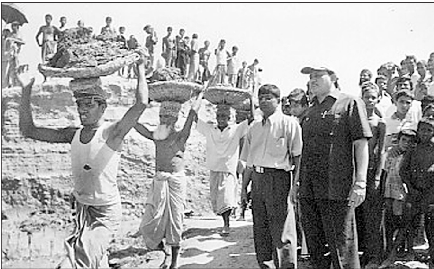
A great job done together...People of Masterpara and Fakir Para villages in Shadullapur giving final touches to the newly dug canal to protect the area from erosion and flooding by Ghagot river. Gaibandha DC Tapon Chandra Majumder (wearing a cap) inaugurated the canal last week.
