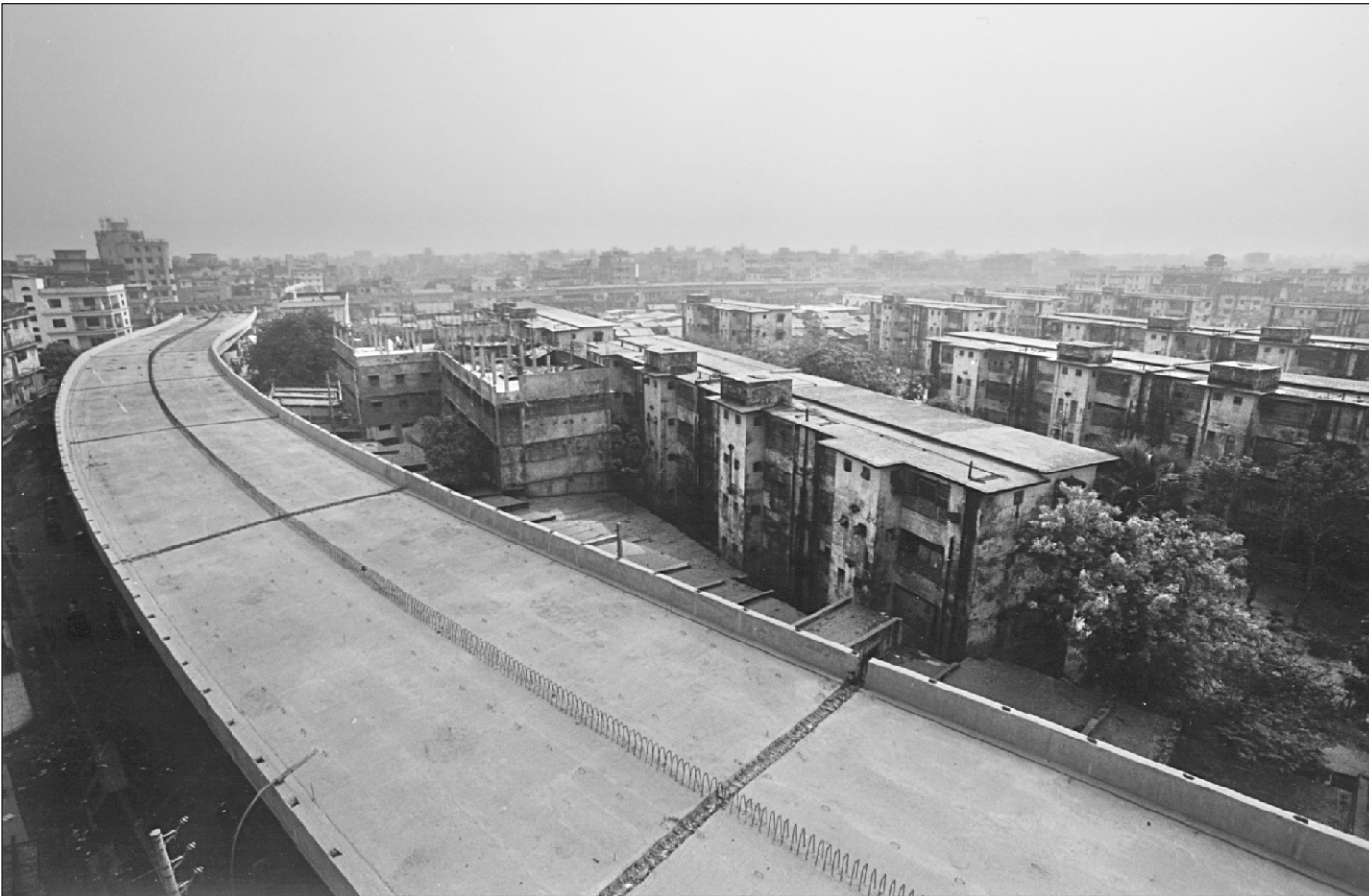
khilgaon flyover project is limping although over 70 percent of the total work have been finished.
