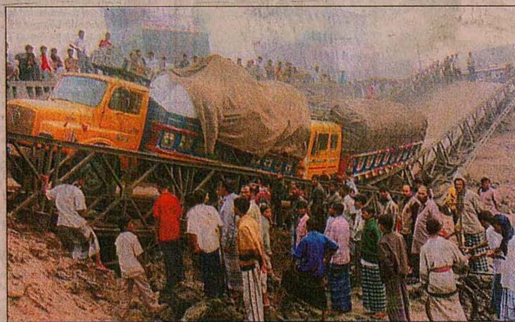
The Bailey Bridge at Sayedabad collapsed at 3:45am yesterday under the weight of these two heavy trucks. No one was wounded in the incident that reportedly caused the state exchequer Tk 5 lakh in losses.
