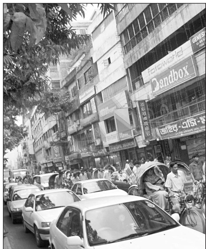
Ribbon development along New Elephant Road causes severe traffic congestion.
