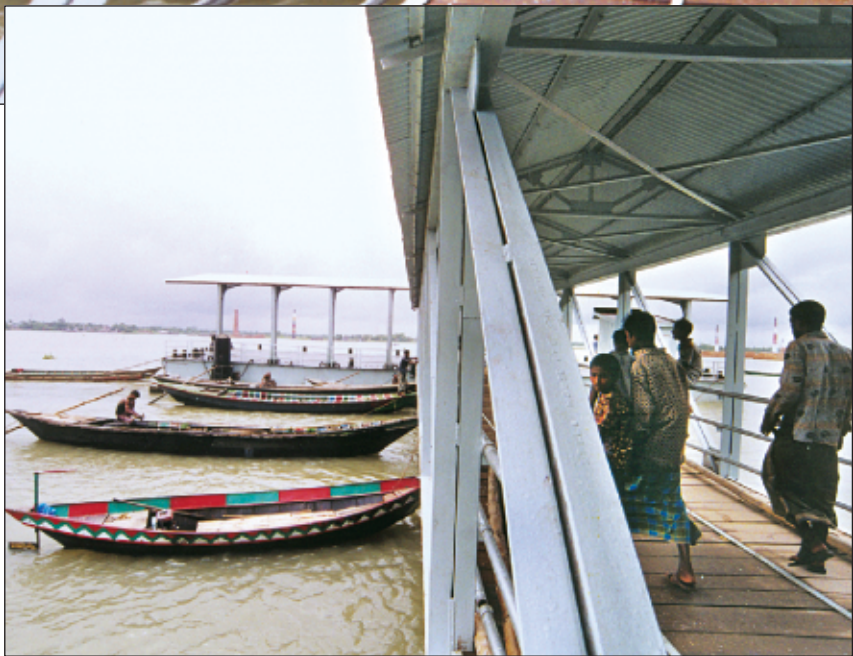
Above and top: The new BIWTC pontoon at Basila, part of the city's circular waterway project now being delayed. Above right: A capstan on the pontoon remains unused by boats plying the Buriganga.
