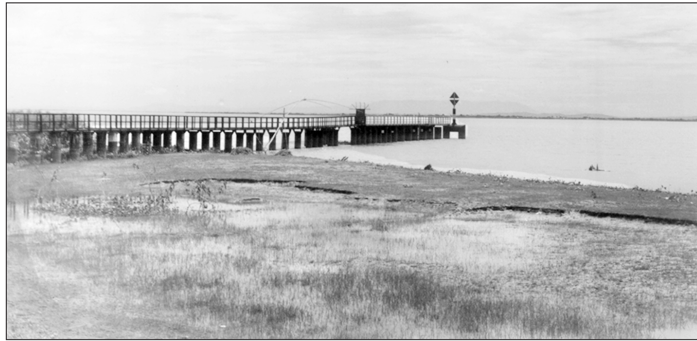
Loss of public money ... this is one of six groynes built in Dhutichara area on the west bank of the Brahmaputra under the Flood Action Plan (FAP) at a cost of Tk 80 crore to protect the bank from erosion. But soon after its construction, over one kilometre area in the downstream along the bank vanished, rendering several thousand people homeless.
