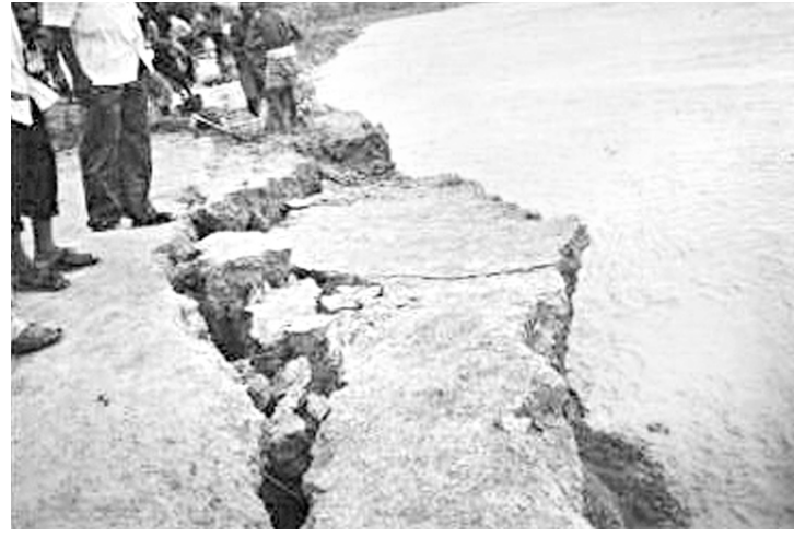
(Left) Unabated erosion of Bhola town protection embankment by the Meghna and (left) sandbags being dumped by local people to check erosion.
