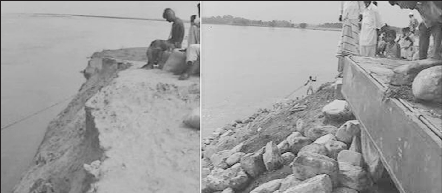
(Left) Water gushing through the breach in the Teesta embankment at Dalia in Nilphamari and (right) boulders being dumped by the authorities to stop further erosion. The photos were taken on Saturday.
