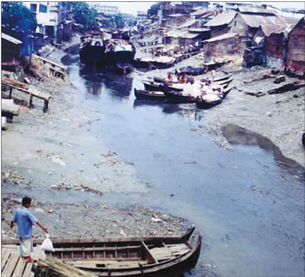
Chaktai canal, the backbone of drainage system of the port city, has silted up to such an extent that even a little shower causes severe water-logging.
