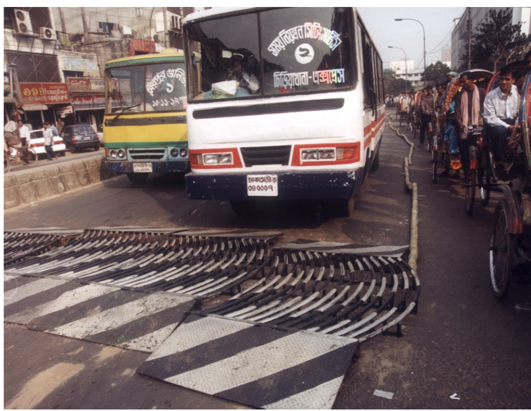
PHOTO: STAR An innovative bump to prevent rickshaws from jumping lanes at work in front of the Jatiya Press Club. An engineer developed and demonstrated the bump yesterday.
