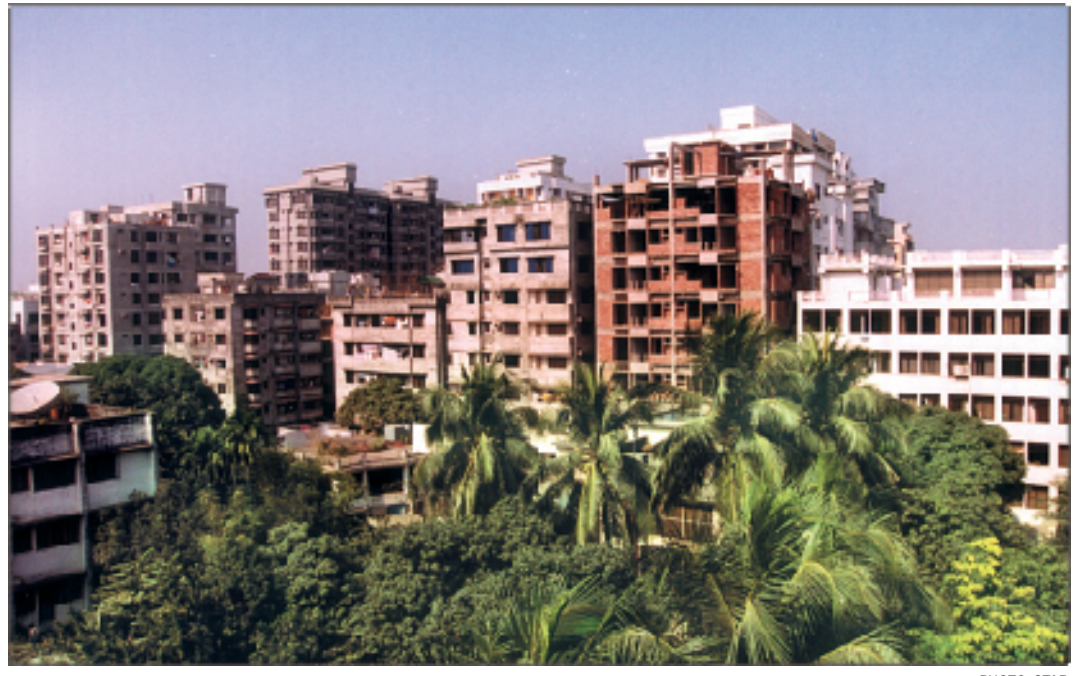
High-rises tower over Dhanmondi, a city residential area where only six-storey buildings are permitted. The buildings have been raised in gross violation of construction rules.
