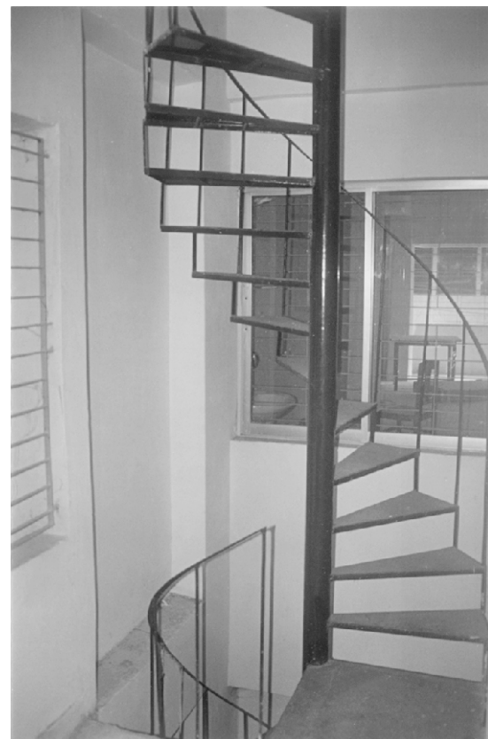
Fig. 4: Western Tower Apartment: A circular staircase designed as fire exit with a window opening towards it.
