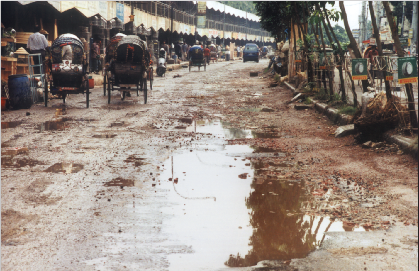
Katabon Road, an important link between the Elephant Road and Nilkhet, has taken a dilapidated look with potholes. The roadside petshops constantly drain out refuse on the road worsening the situation.
