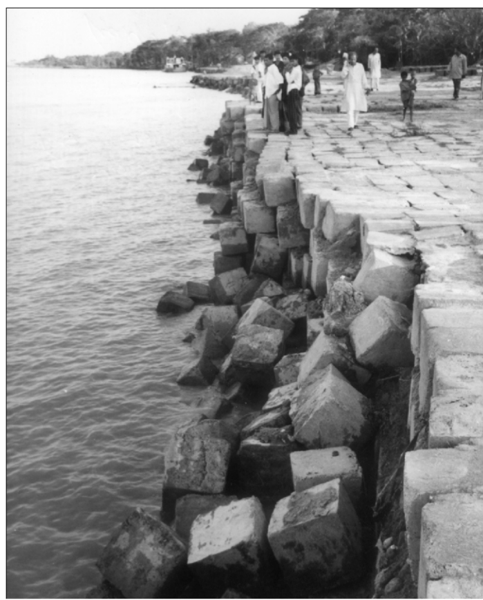
Unabated erosion in Bhola by the Meghna despite placement of boulders along the river bank. Erosion has taken a serious turn here in recent days.
