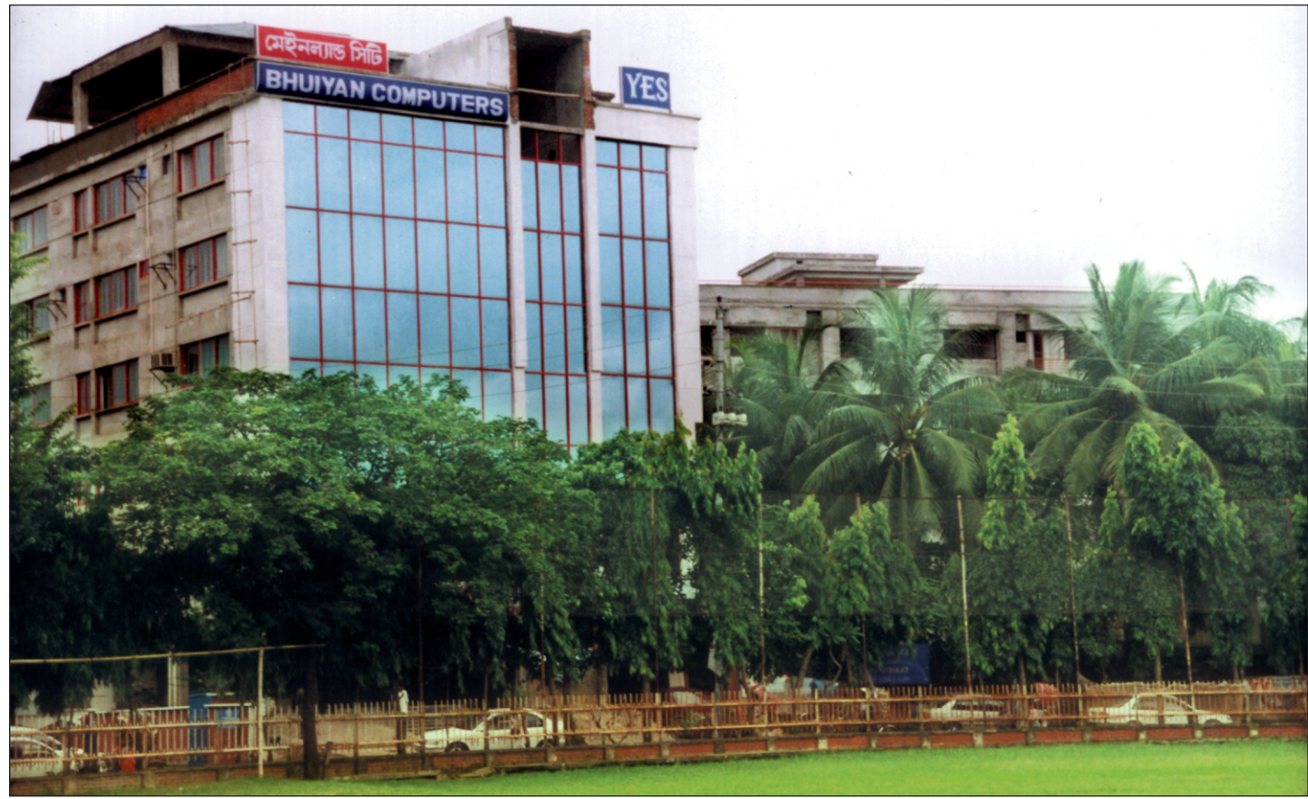
PHOTO: STAR An illegally built six-storied commercial complex stands high on the western side of the Dhanmondi playground -- an example of how the city's residential areas lose their liveable qualities to the commercial conversion of plots.
