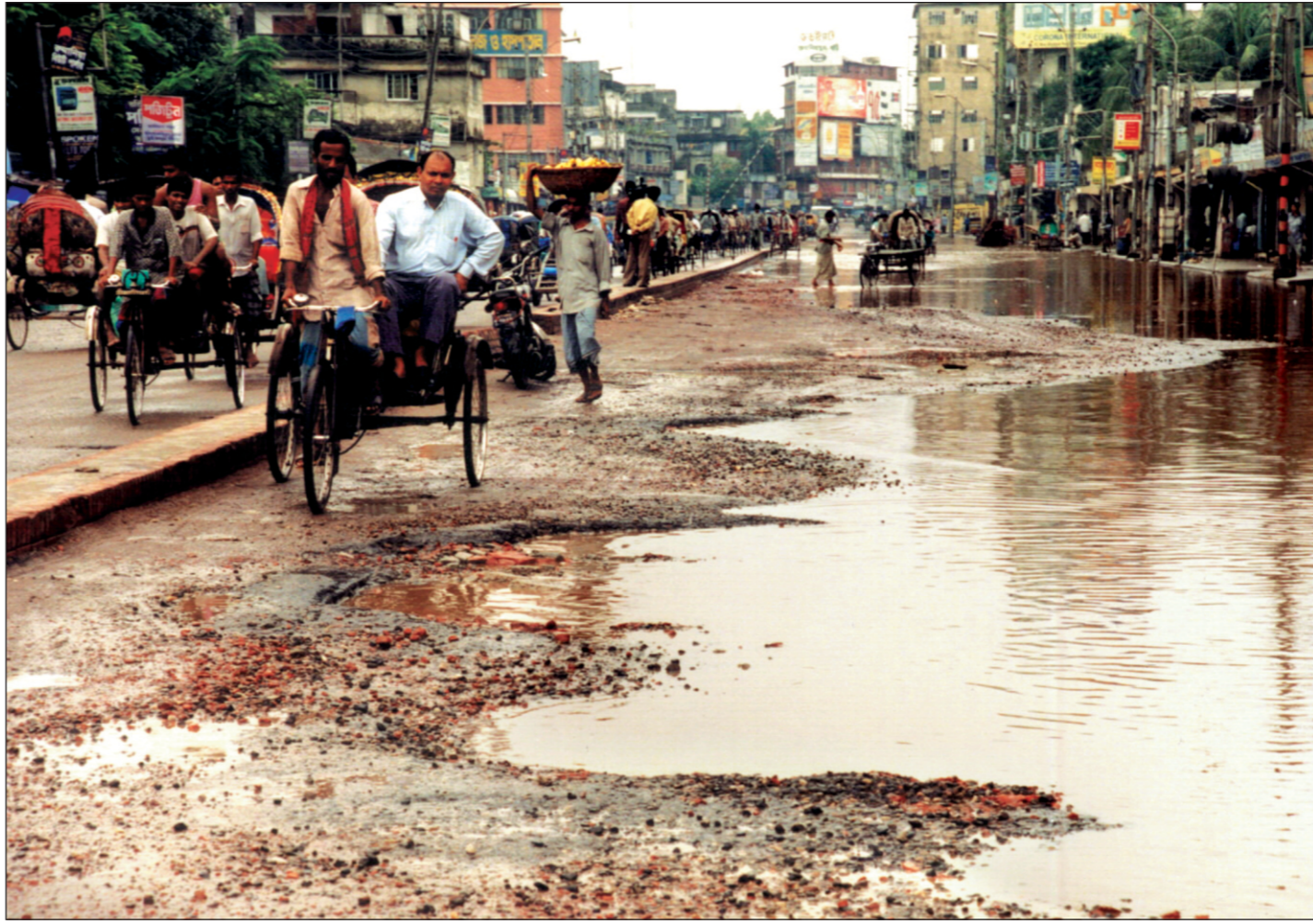
Call it a road... the Malibagh Road, full of potholes with stagnated rainwater, aptly sums up the miserable conditions of major thoroughfares in the city. The Dhaka City Corporation (DCC) remains blissfully unaware.
