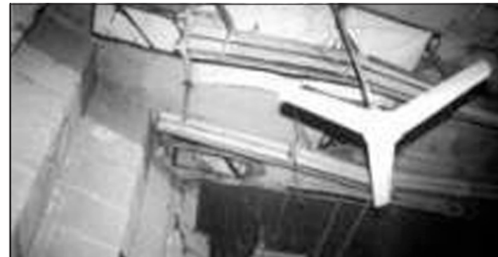
Another view of Guide House ceiling
