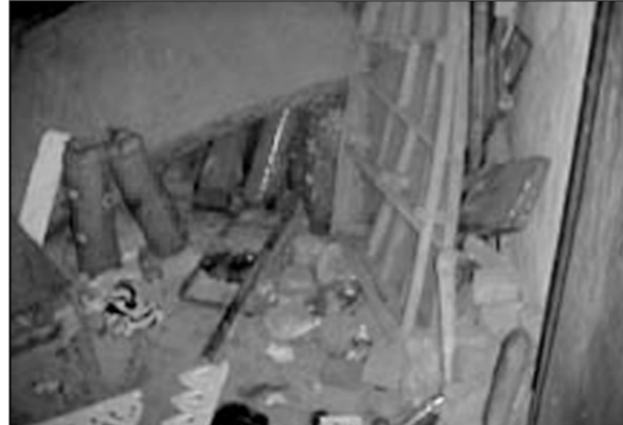
Fire extinguishers out of order at Public Library auditorium
