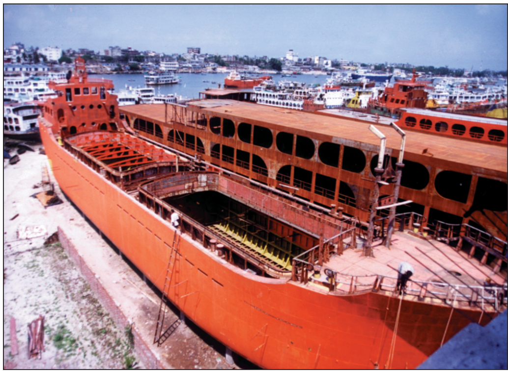
Vessels are being built at a makeshift dockyard.
