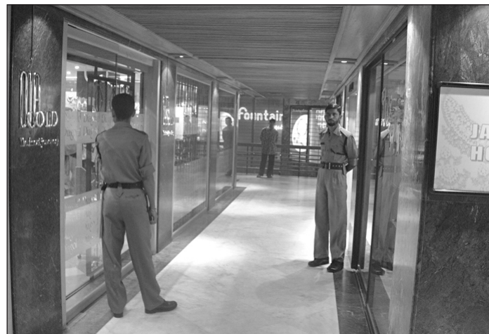
Too much use of combustible material in interior.
