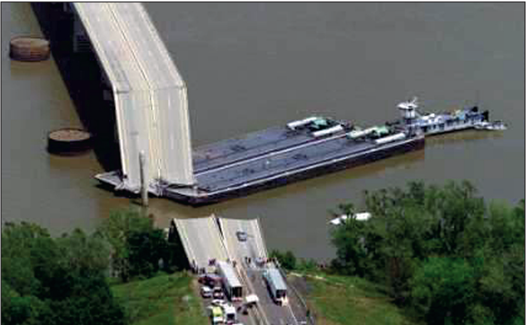
A large span of Interstate 40 in Oklahoma lies in the Arkansas River on Sunday after a barge hit the moorings and pitched as many as 12 vehicles into rain-swollen waters below the heavily travelled highway bridge. The 500-foot section of the bridge gave way after being rammed by an empty oil barge.
