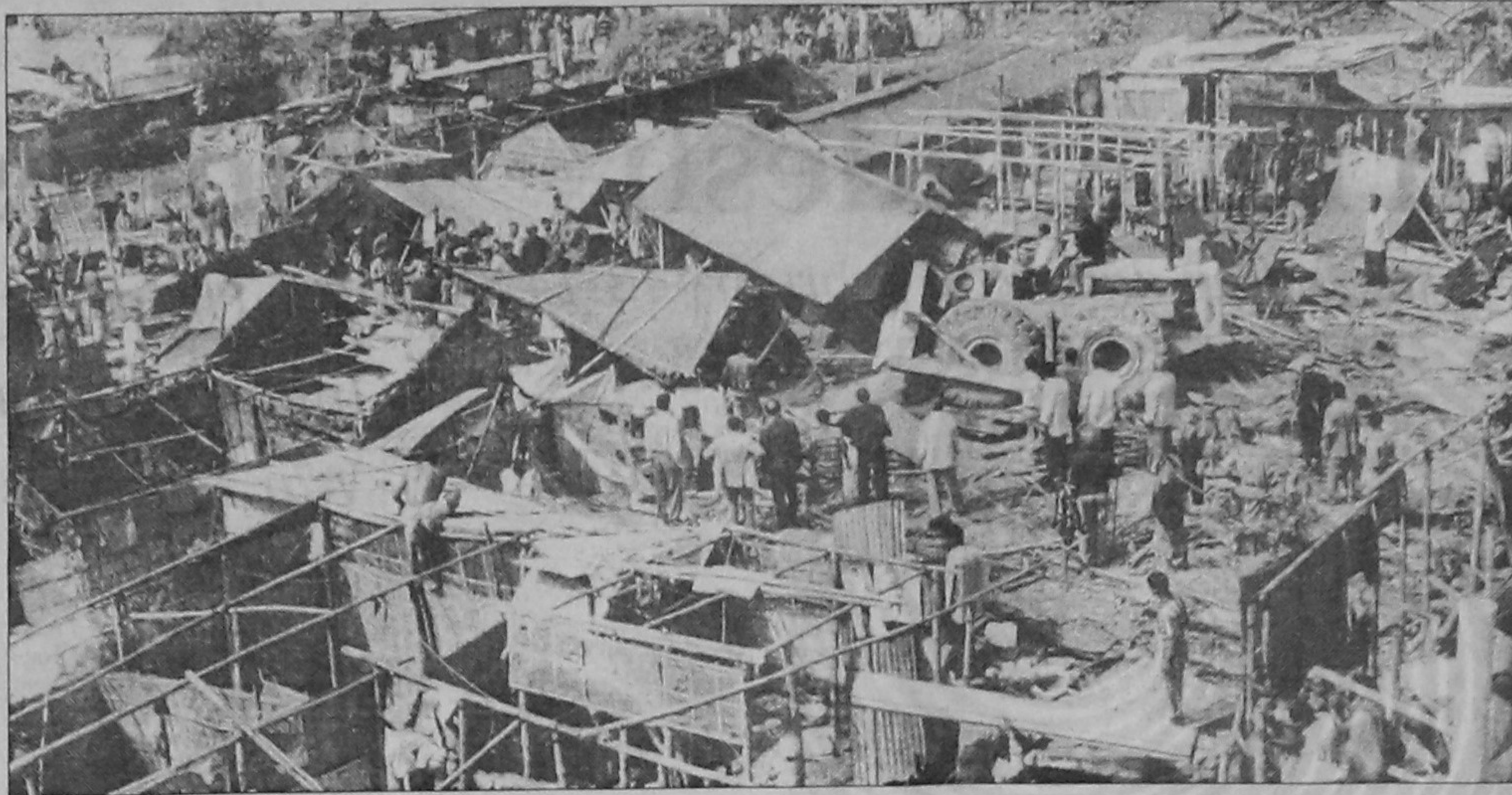
Public Works Department demolished a slum at Agargaon in the city yesterday.
