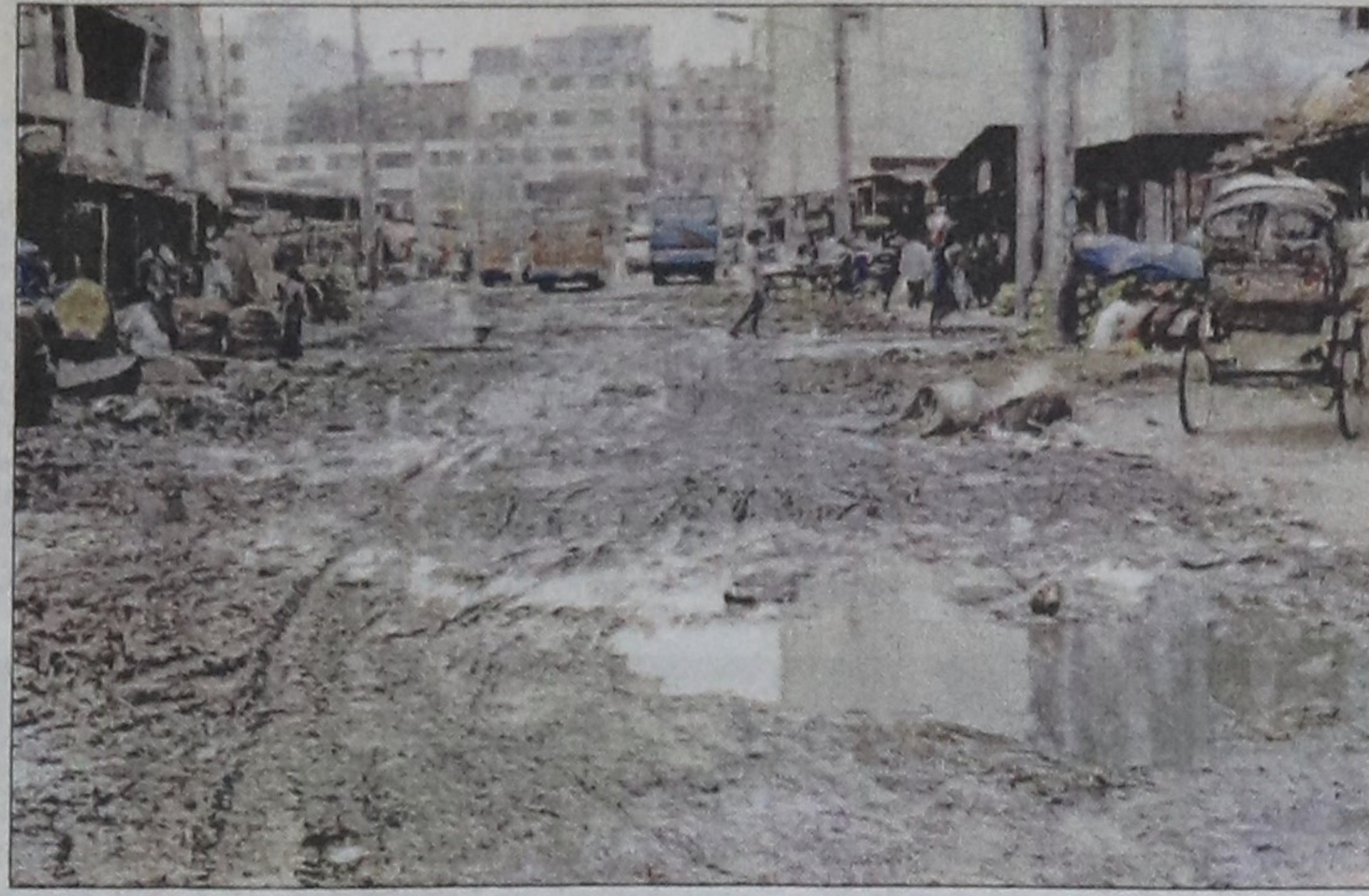
PHOTO STAR This road at Karwan Bazar has been littered with filth and riddled with potholes for long, but the authorities seem indifferent to the woes of the road users.
