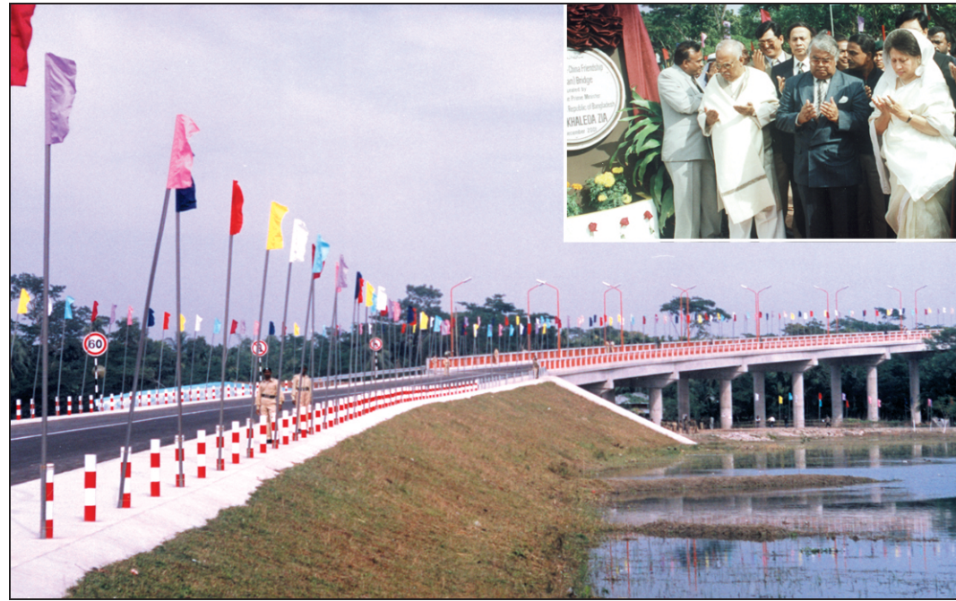
The Fifth Bangladesh-China Friendship Bridge over Gabkhan river in Jhalakathi was opened to traffic yesterday. Prime Minister Khaleda Zia offering munajat after inaugurating the bridge (inset).
