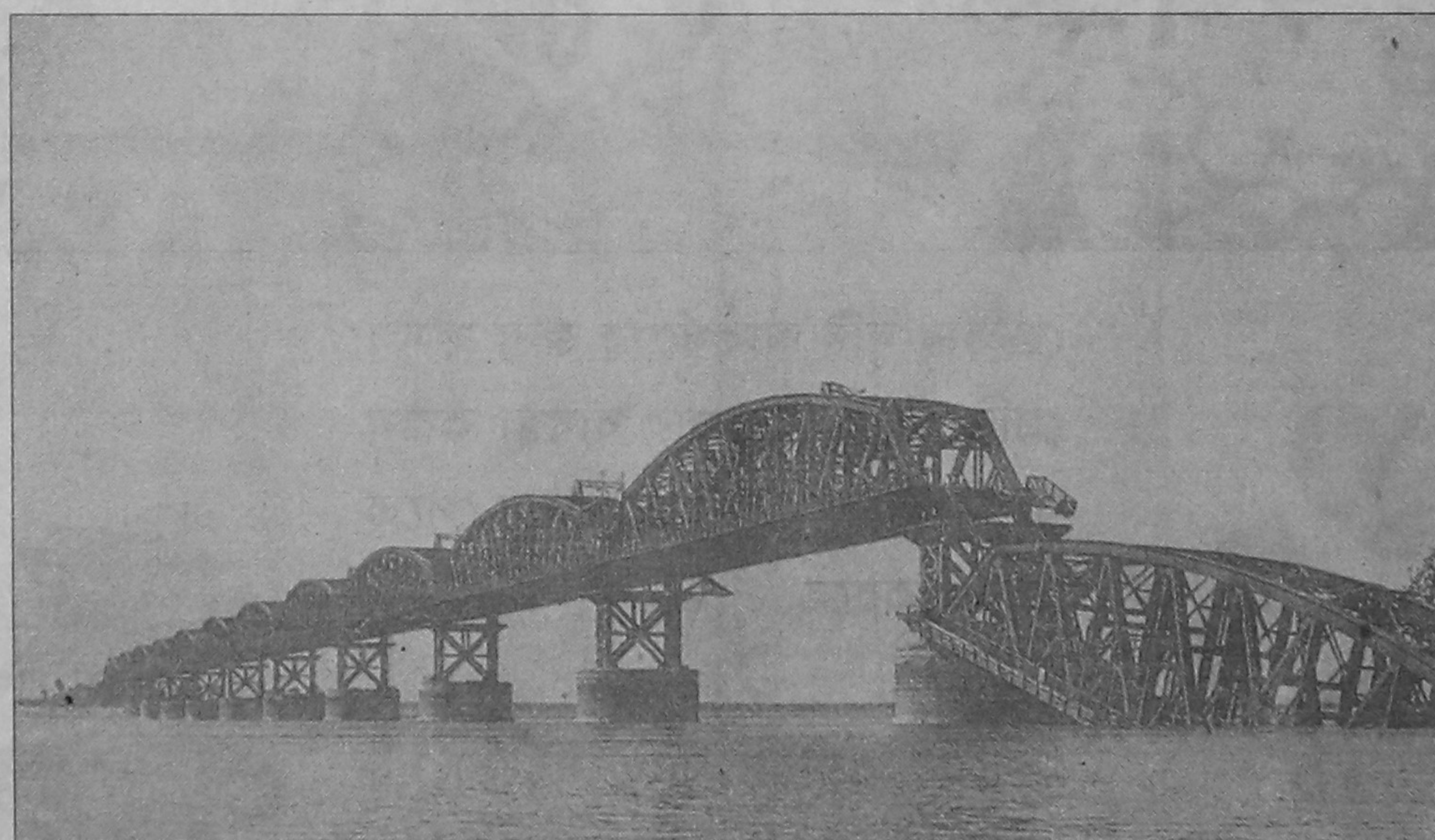
Devastated Hardinge bridge
