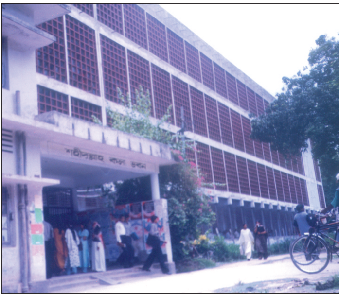
Shahidullah Arts Building, one of the overcrowded academic buildings of Rajshahi University.
