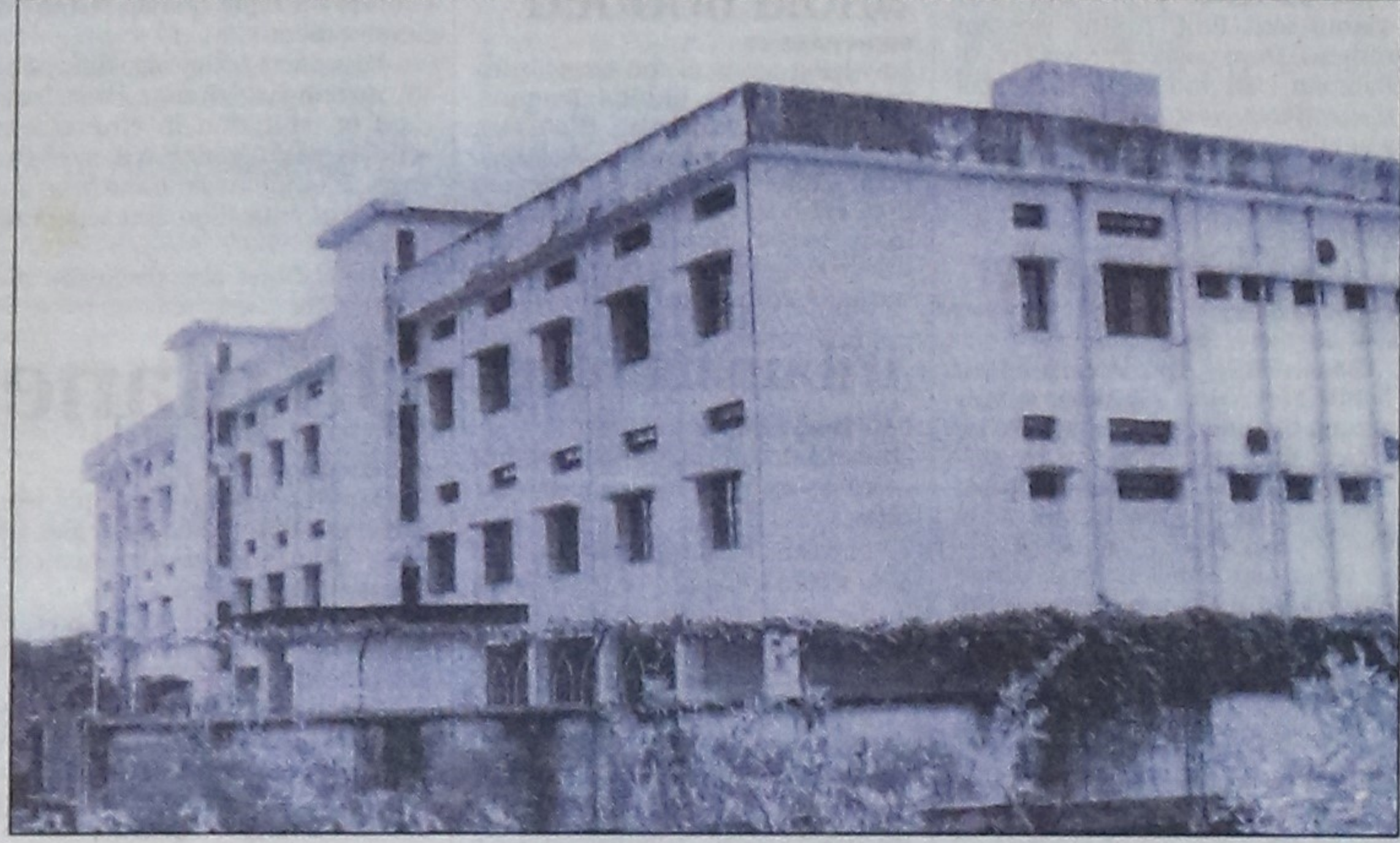
The 20-bed hospital at South Charaicha under Char Fasson upazila in Bhola
