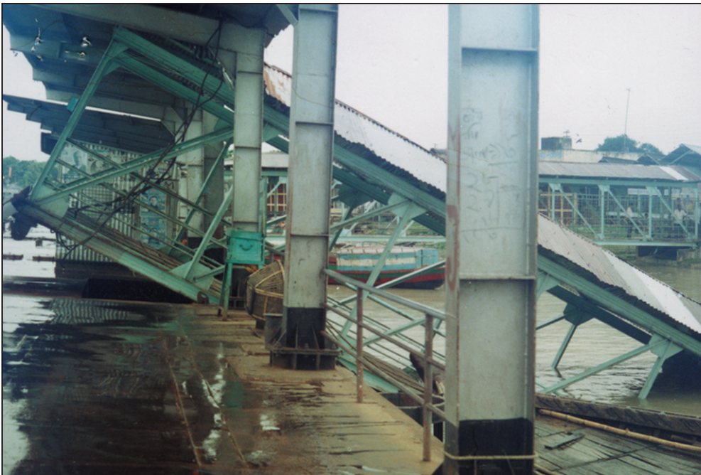
Part of the BIWTA terminal at Chandpur crumbled due to river erosion (left) and the onrush of water of the Meghna and the Dakatia brought hotels and shops in the terminal area on the verge of collapse (right).
