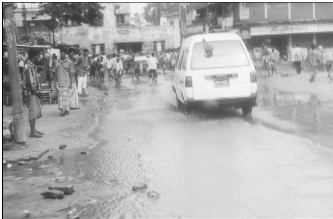
Jhenidah Post Office area in Jhenidah town remains clogged, waterlogged even after moderate rains due to faulty drainage system. But who cares?
