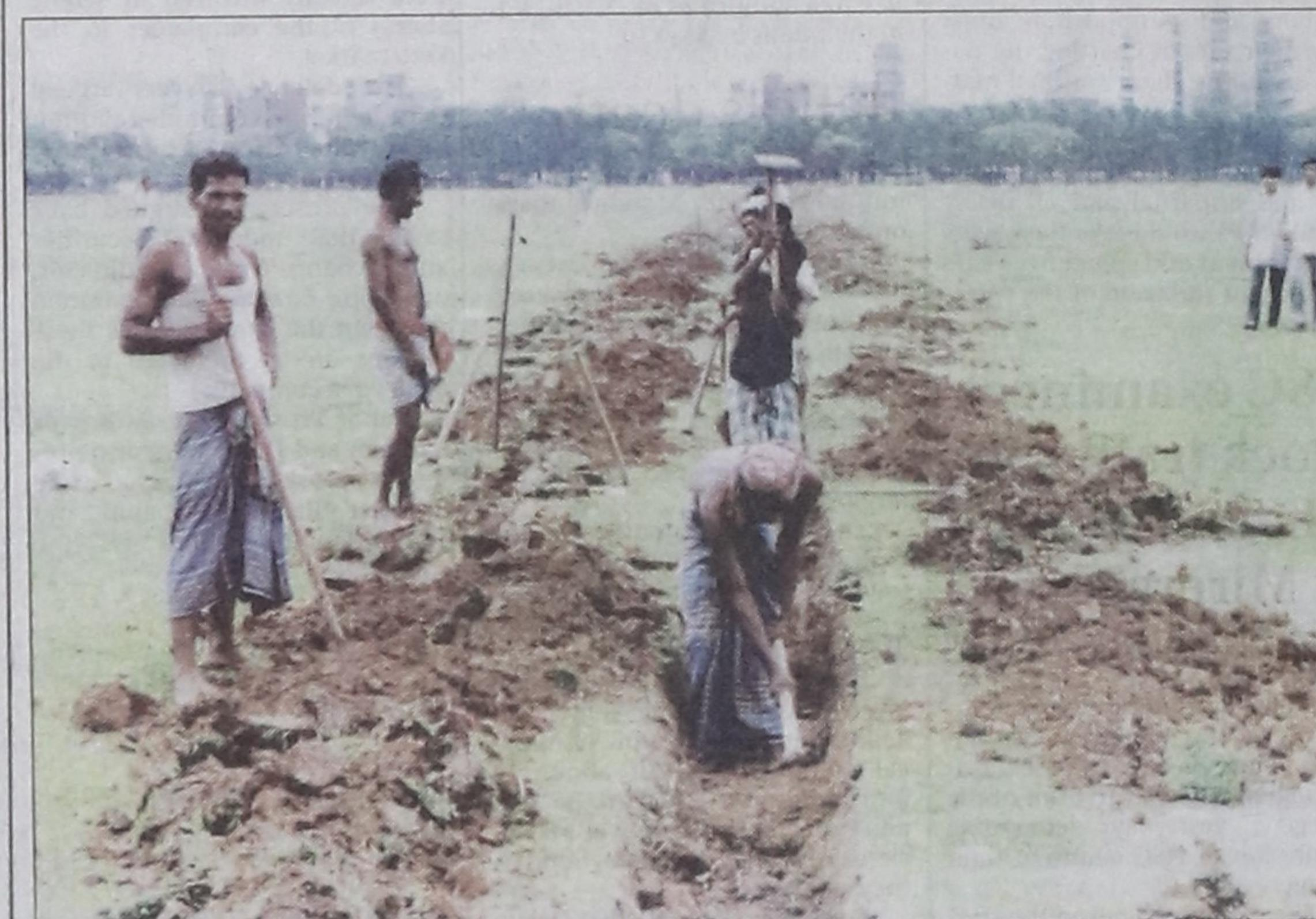
Work is underway on the southern plaza of the Sangsad Bhaban to replace old water pipes running at five different places on the entire length from east to west of the open space.
