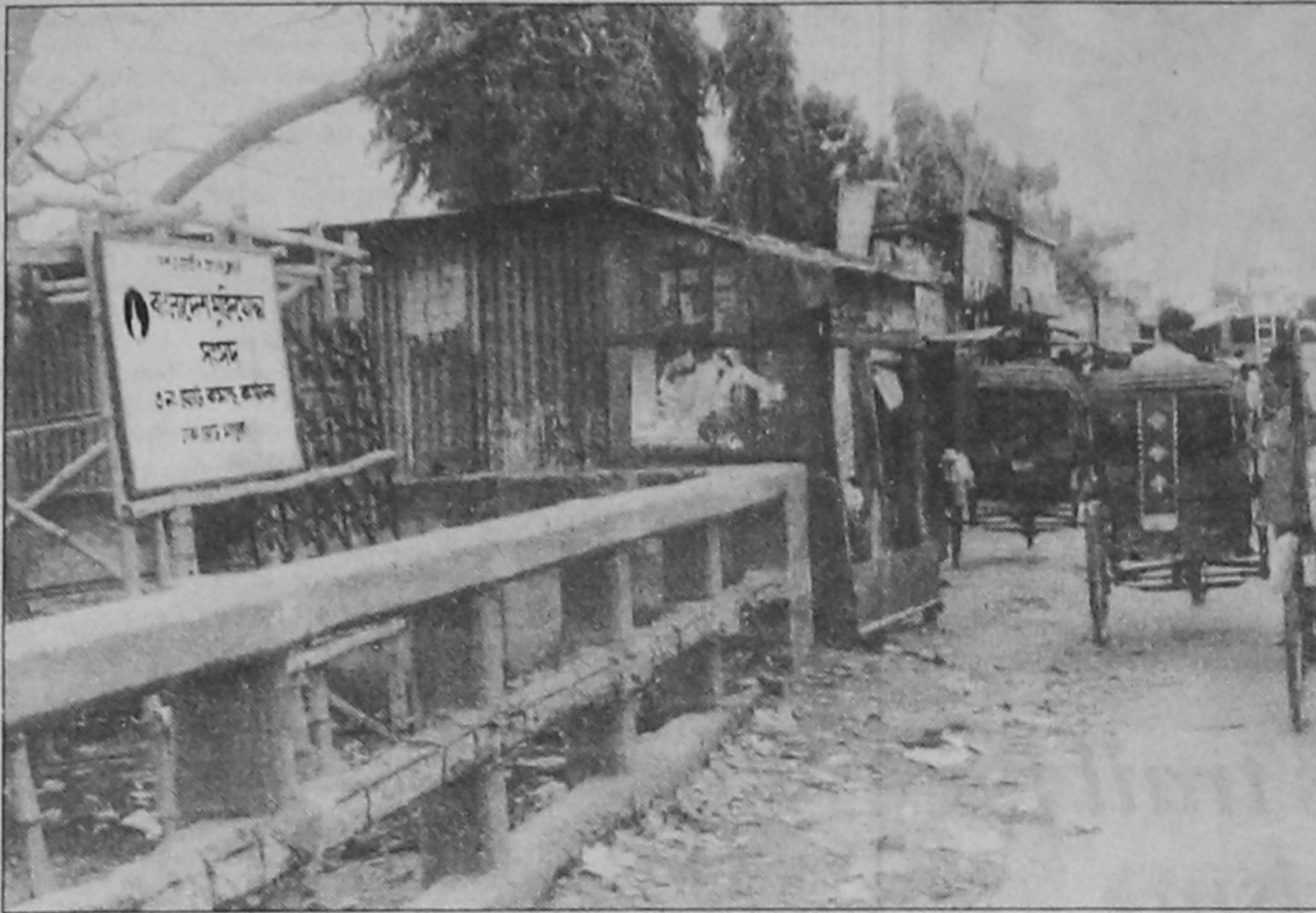
Picture shows unauthorised structures at Dhaka Road Bus Stand in Magura. These days the district has been witnessing the sprouting of such structures on both sides of the roads and highways.
