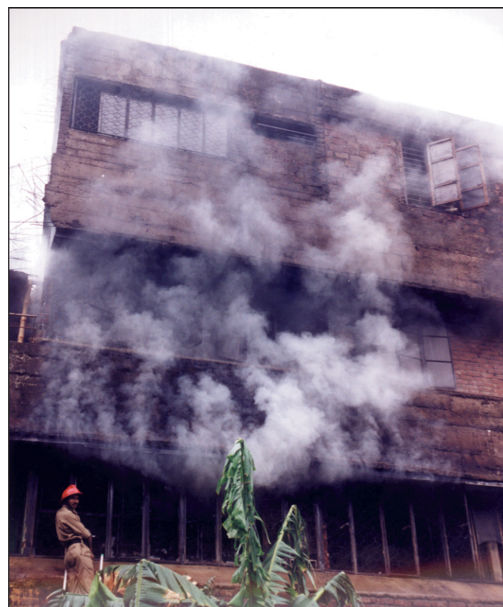
Fire at a Bata warehouse at Lily Plaza near Mouchak market in the city gutted shoes, leather worth Tk 5 lakh yesterday.
