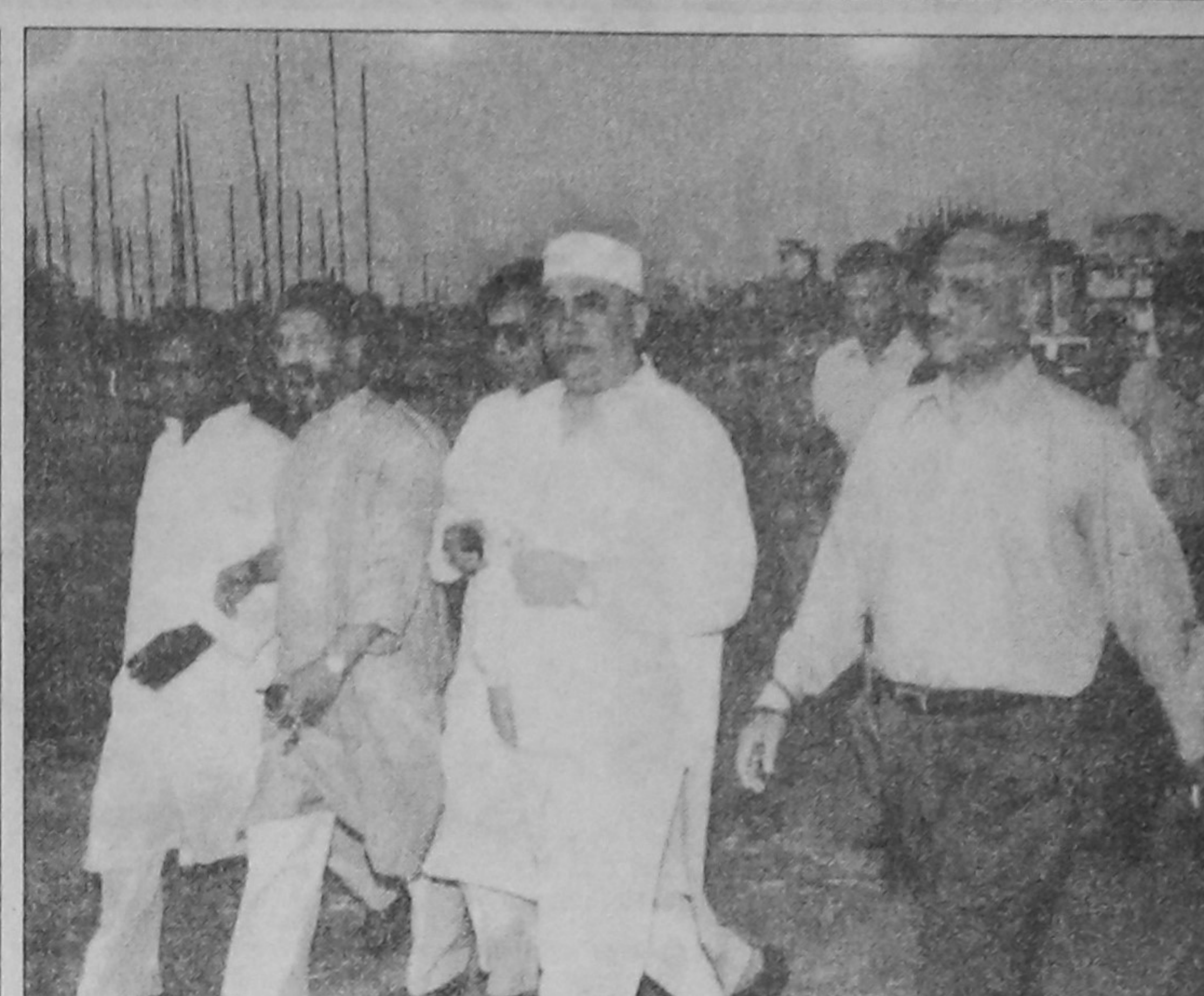
State Minister for Youth and Sports Obaidul Quader (R) and Bangladesh Cricket Board president Saber Hossain Chowdhury inspecting the construction work of the National Stadium at Kamalapur-Mugdopara in the city on Tuesday. It is expected that the first phase of the construction work to make the football stadium fit for play will be finished by June this year.
