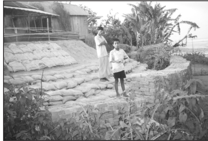
The Water Development Board (WDB) authorities have constructed a pucca flood protection embankment along Shimla area in Sirajganj. The local people have been planting saplings of various fruit bearing trees and flowers along the embankment area. --Starphoto
