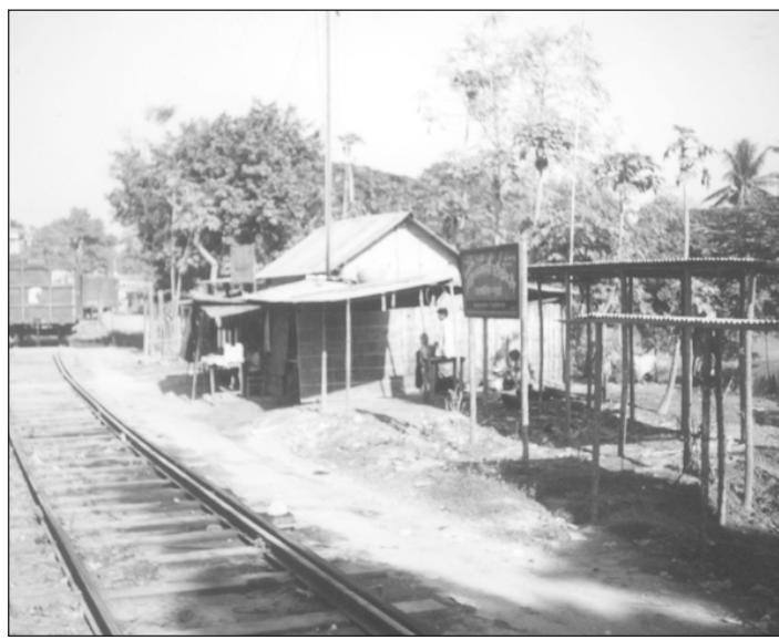
A section of influential people build many illegal structures on railway lands in Sirajganj Bazaar Railway Station area. ---Star photo
