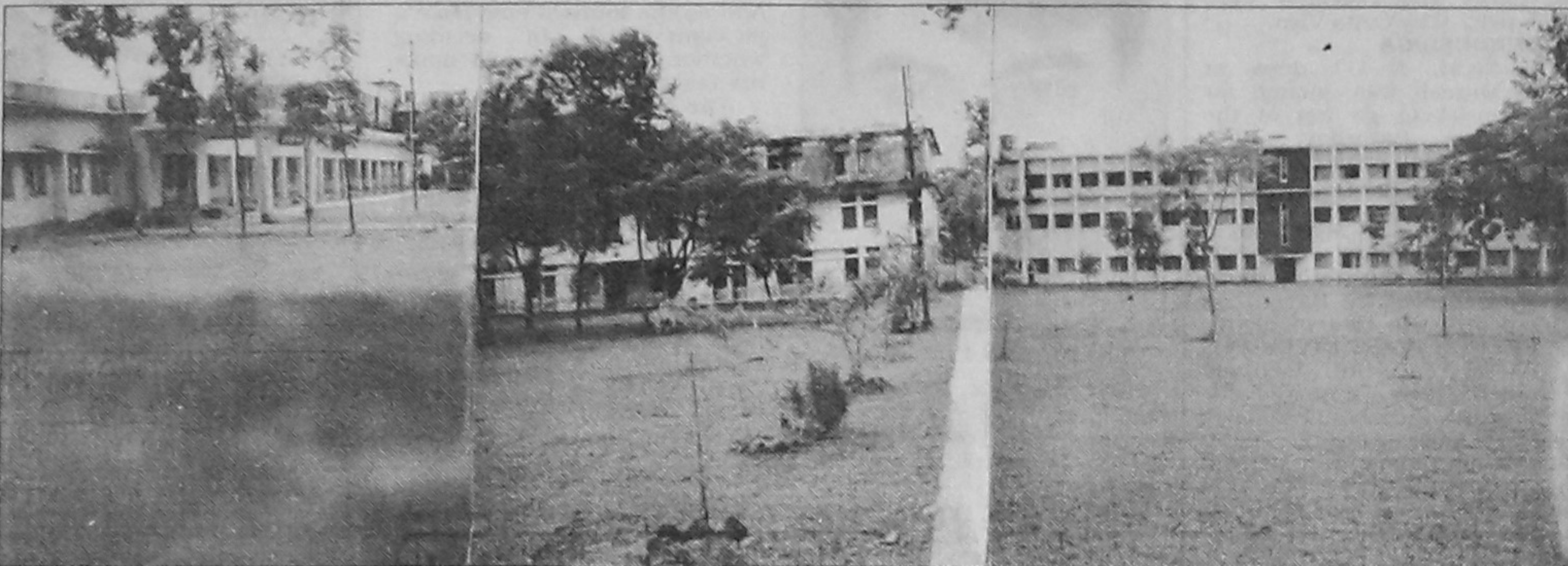
(Far left): Partial view of the main building of Netrakona Primary Training Institute (PTI) (Middle) Female hostel with no boundary wall where boarders feel insecure due to frequent harassment by local vagabonds (Far right) Male hostel with cracked roof where boarders suffer a lot even in slight rain. --Star photo
