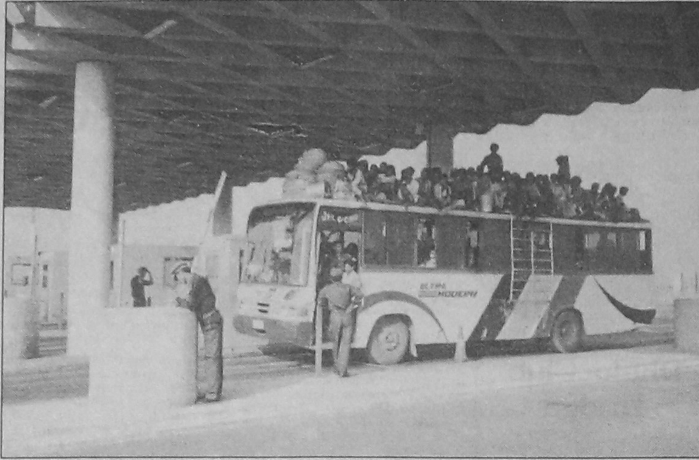
Travelling on roof-tops of highway buses going on unabated despite some serious bus accidents including the worst-ever highway disaster on April 29 in Sirajganj district along this northern highway. This photo was taken recently on Bangabandhu Jamuna Bridge. —Star photo
